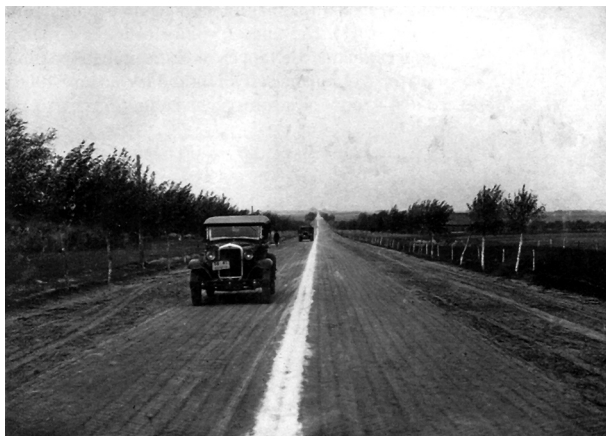
Fig. 4. Gomel-Kalinkovichy, one of the first automobile roads in Belarus. The photo of the 20s, XX century
